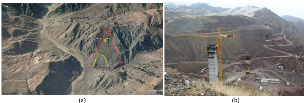
Figure 1 - 370 km landslide a) Image is taken from Google Earth from the landslide area, the yellow part of the smaller and newer landslide that has occurred in the displaced mass. b) Picture of Bridge No. 12 to the northeast
